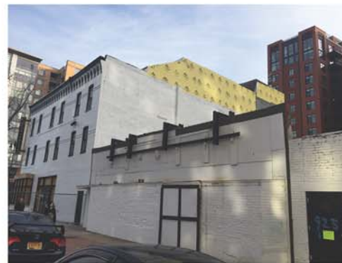
EXISTING BRICK FACADES
