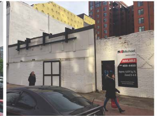
EXISTING BRICK FACADES
