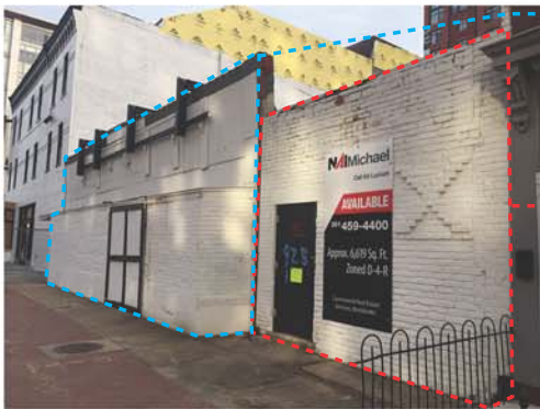
EXISTING BRICK FACADES
